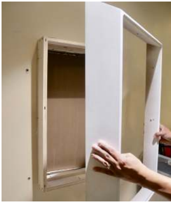
Attach outer Frame on inner Frame. Hold tight against wall when attaching, to minimize gaps on side next to wall.
