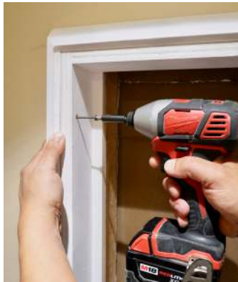
Attaching inner part of Frame to outer Frame. Four screws, two per side.
