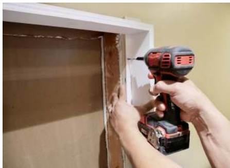
Attaching Frame to wall and 2"X4" stud. two screws on each side (top, middle and bottom).
