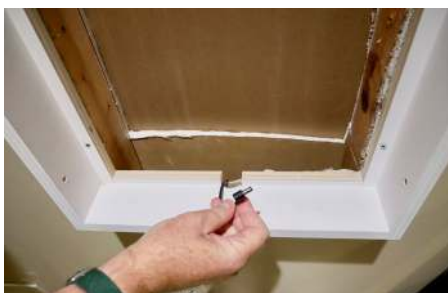
Pull wire up from wall through wire hole in Frame bottom.
