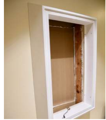
Complete Frame attached to wall, winder power wire on bottom part of Frame.
