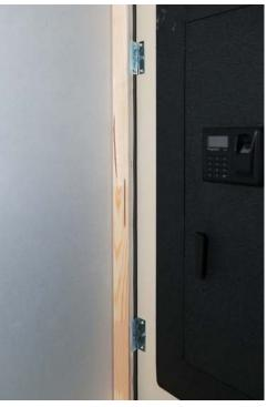
We mount the hinges on the back of the wood frame and to the wall (see photo). If there is a stud in the wall to attach the hinges to, great; if not, just put some light anchors into the wall for the hinges to screw into.
